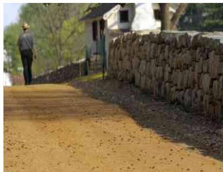
John Hennessy, chief historian of Fredericksburg & Spotsylvania National Military Park, walks along a restored section of Sunken Road in Fredericksburg. The re-created Civil War-era road is a combination of dirt, gravel and clay. (photo courtesy Fredericksburg Free Lance-Star)
