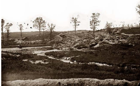
May 1865 view of the interior of the Confederate line at Gracie's Salient, Petersburg. Timothy O'Sullivan took this photograph which was published in Alexander Gardner's Photographic Sketch Book of the War in May 1865. It shows earthworks, bombproofs on the right, chevaux-de-frise and hurdle revetments and Poor Creek. (Library of Congress)
