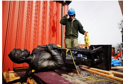
NPS monument preservation specialist Lucas Flickinger prepares to connect a crane harness to the figure from the 121st New York Infantry monument. Photo by Shane Dunlap, The Evening Sun
