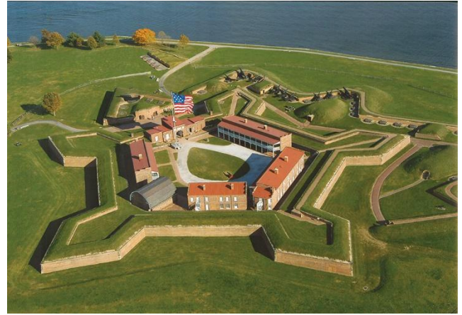
Fort McHenry 2400 E. Fort Ave.
