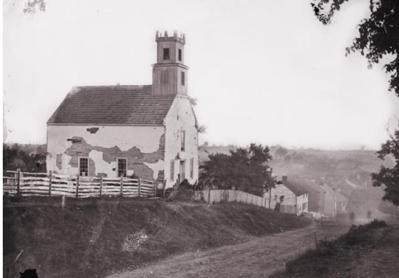
Union artillery shells badly damaged the 1768 Lutheran Church on the east side of Sharpsburg. (Library of Congress)
