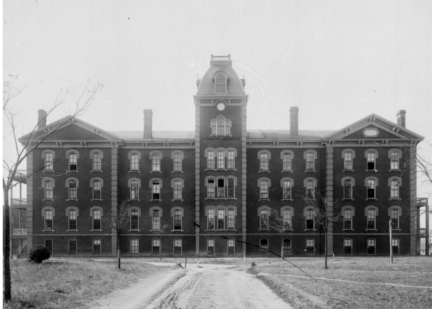
Shaw Hall, a building at the historically Black university that Buss helped establish Public domain via Wikimedia Commons
