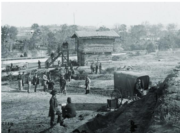
This two-story blockhouse was erected in Arlington Heights, Va., just outside Washington, D.C. It was similar in style to the blockhouses Dodge became famous for constructing along the Mobile & Ohio Railroad to defend against cavalry raids at vulnerable bridges and train stations. (Library of Congress)
